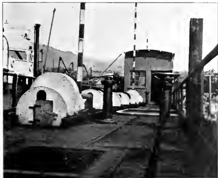
Above—View of the deck of the starboard wing of the smaller section of dock showing one of the four flood gate valve operating stands, one of the four flapper valve operating stands, the motor house, and the horizontal line shafting driving the pumps. The graduated spars are the water gauges for the pontoon. At right—View looking down on the small section of the dock showing the general arrangement.
